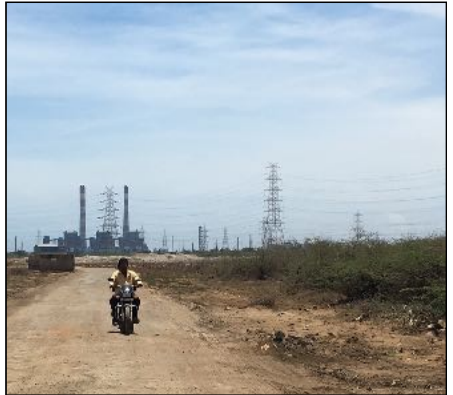
Living in the shadows of the power plant has made life difficult for the residents of Seppakkam
